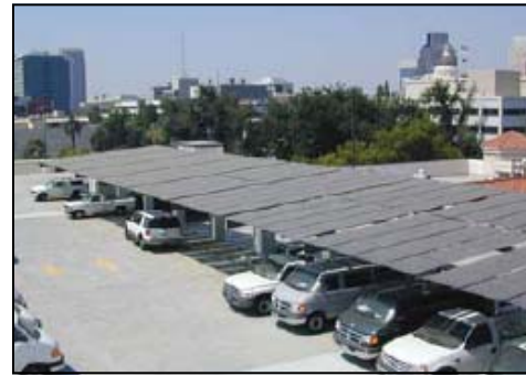
Figure 9-6: A solar power shading device in a parking lot
